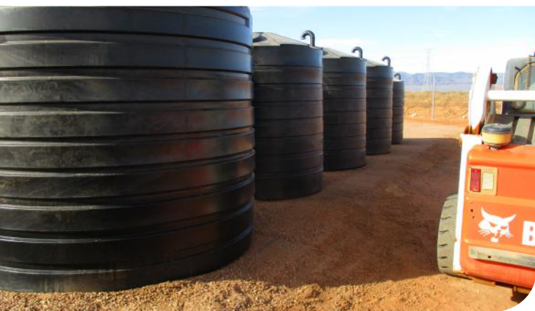
Installation of influent storage tanks
