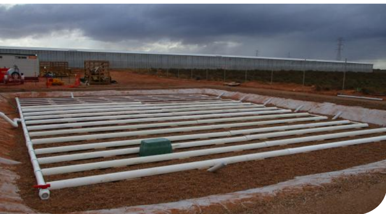
Irrigation pipework installation
