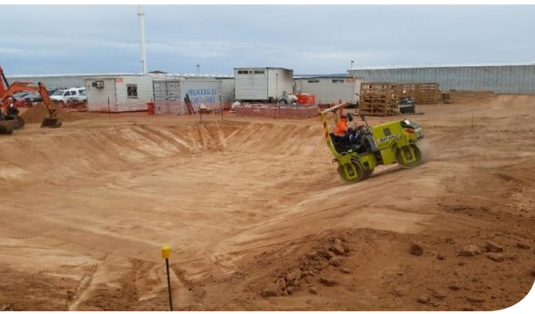
Earthwork construction of basin
