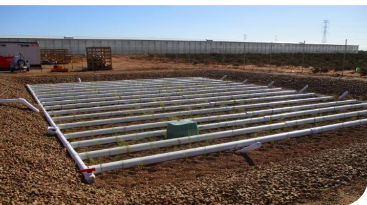
Constructed system showing partial regrowth
