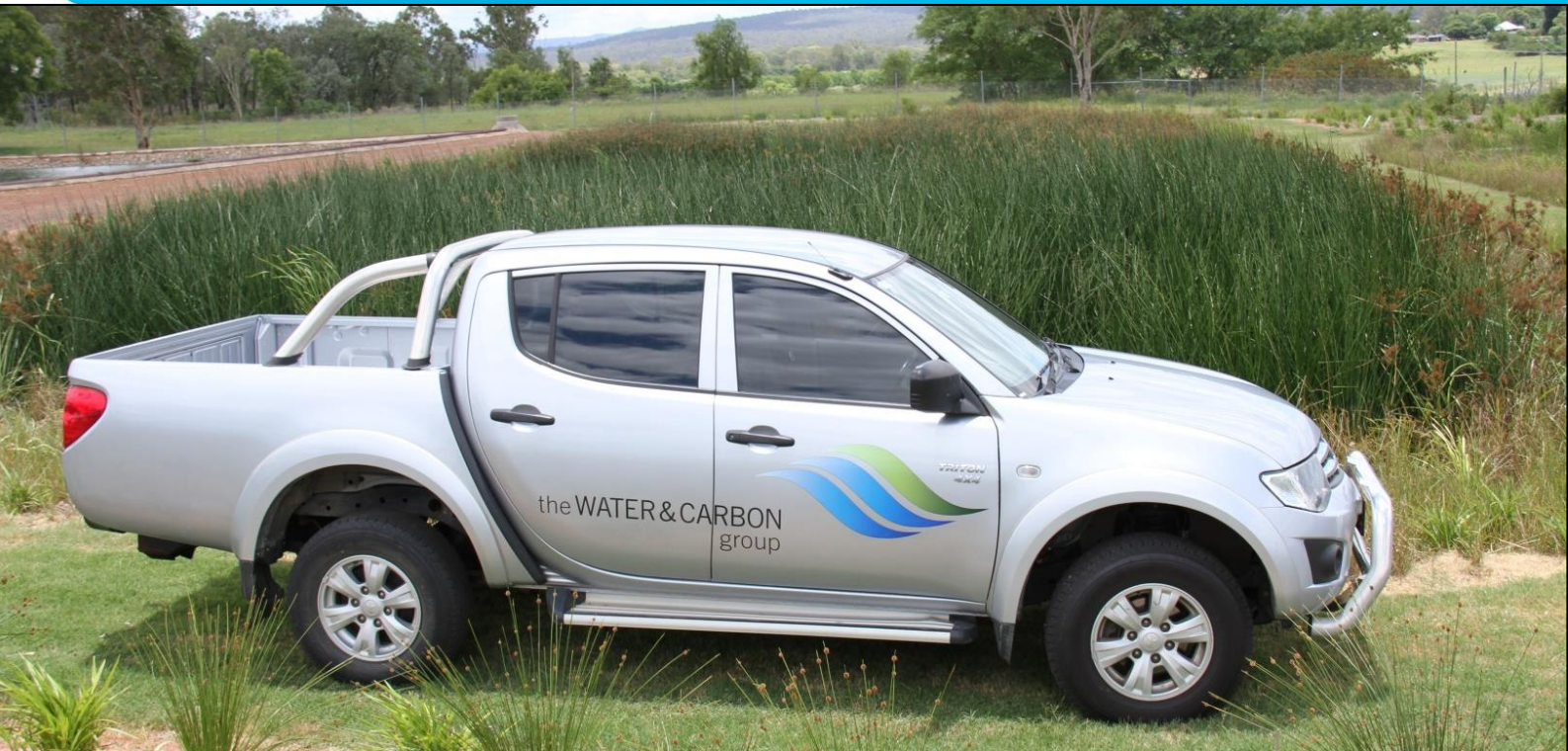
Helidon WWTP – Constructed Wetland
