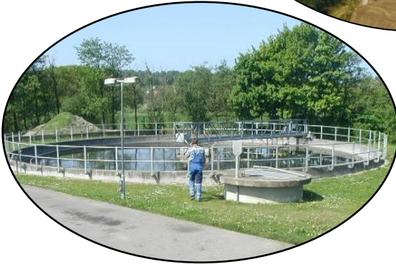
Tisvilde Wastewater Treatment Plant
