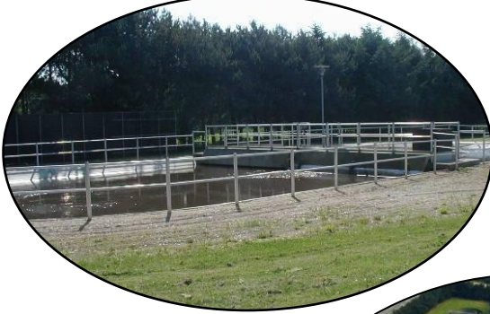
Rågemark Wastewater Treatment Plant
