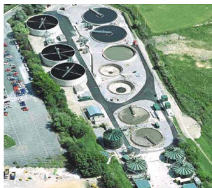
Municipal WWTP Ernesettle, Great Britain
