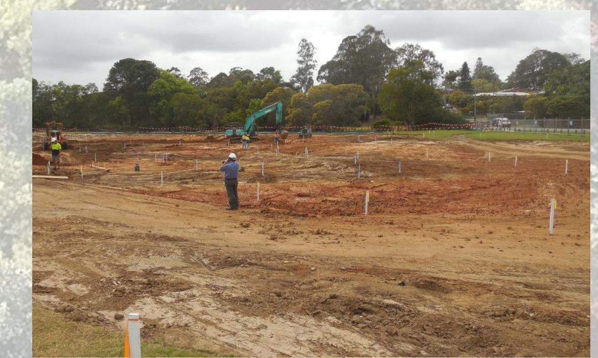
Wetland construction, September 2014
